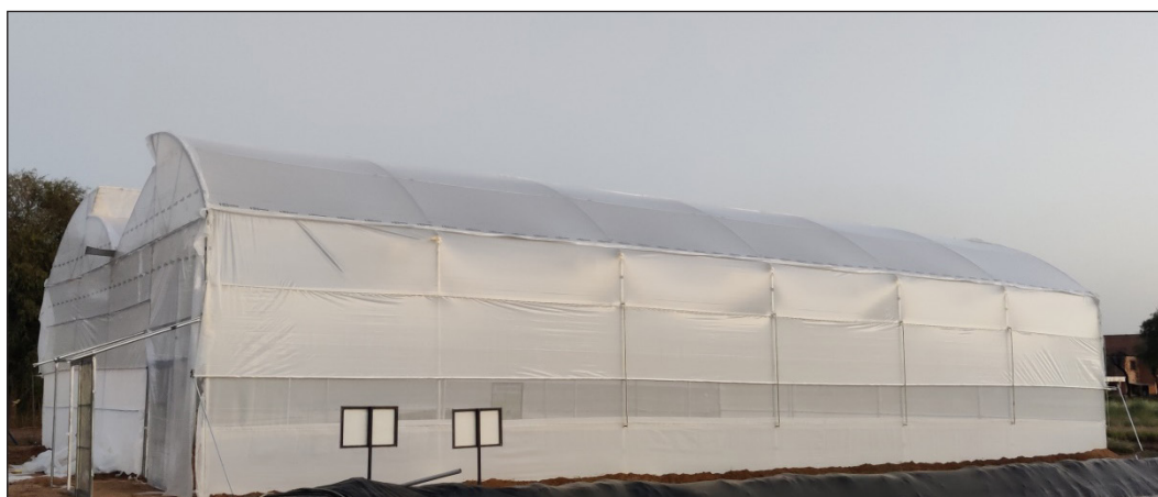
Fig. 3. Naturally-ventilated polyhouse (NVP) erected in the Integrated Farming Cafeteria.
