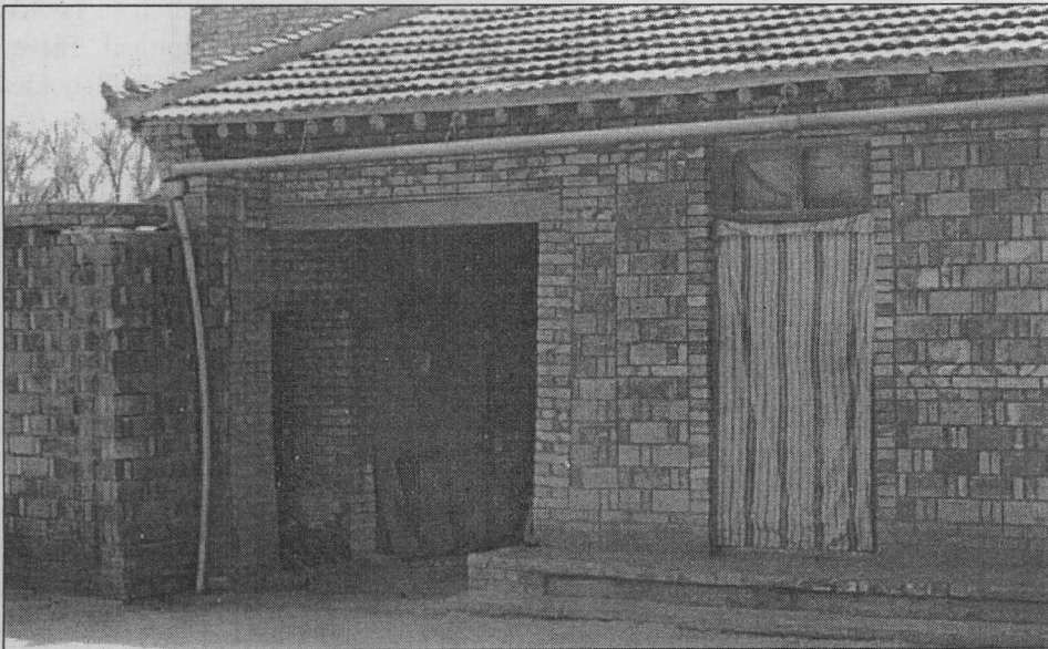
Fig. 8. Rooftops for rainwater harvesting in the Loess Plateau.
