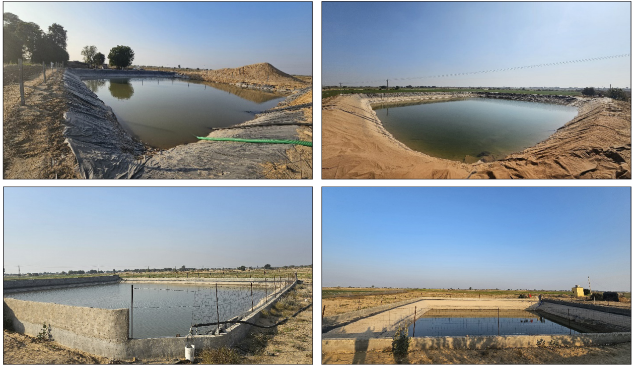
Fig. 2. Types of Diggi structures; Earthen type (upper two) and cemented (lower row) in IGNP command area of Jaisalmer district.
