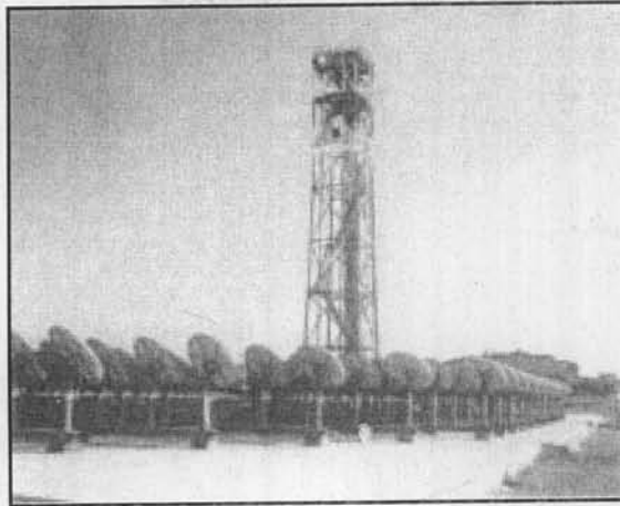
Fig. 14. "La Capanna" experimental solar station at ENEA's Casaccia Research Center (Source: Photo courtesy of ENEA, 1983).
