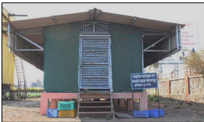
Fig. 2b Onion storage structure
