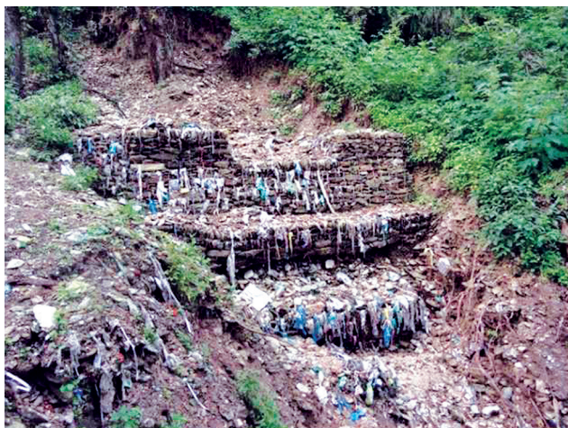
Fig 3 Gabion structure constructed
