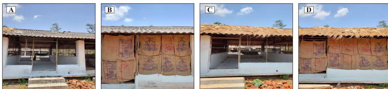
Supplementary Fig. 1. A. Asbestos roof as control (TA); B. Asbestos roof with gunny bags as screen (TAG); C. Modified asbestos with thatched roof (TH); D. Modified asbestos with thatched roof with gunny bags as screen (THG).
