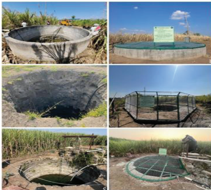
Fig.4. Mitigation measures implemented to prevent accidental wildlife falls; pre-intervention images (a, c, e) depict open wells at high-incident zones, post-intervention images (b, d, f) illustrate successful installation of lids and protective barriers
