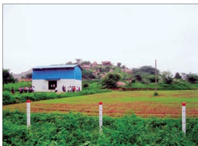
Biomass Bunker (Fodder bank) at Gochar land
