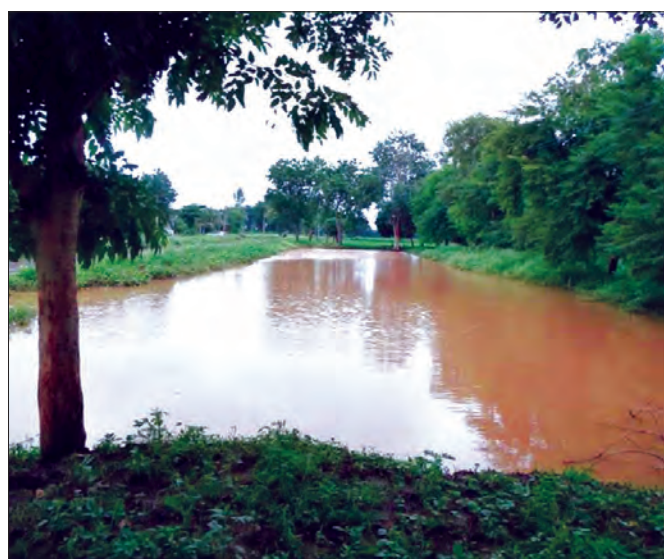
Water harvesting tanks for run-off collection.
