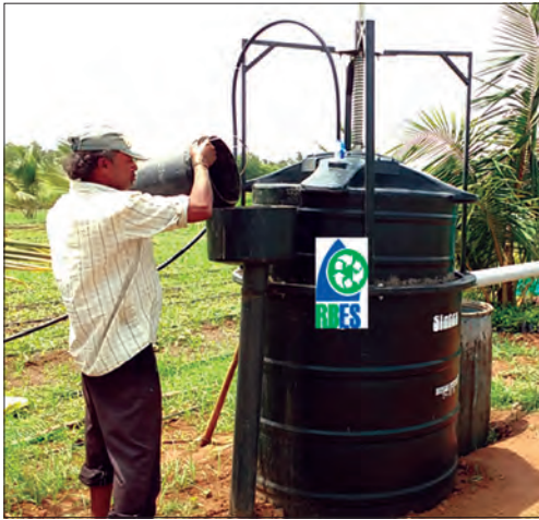
Portable biogas plant
