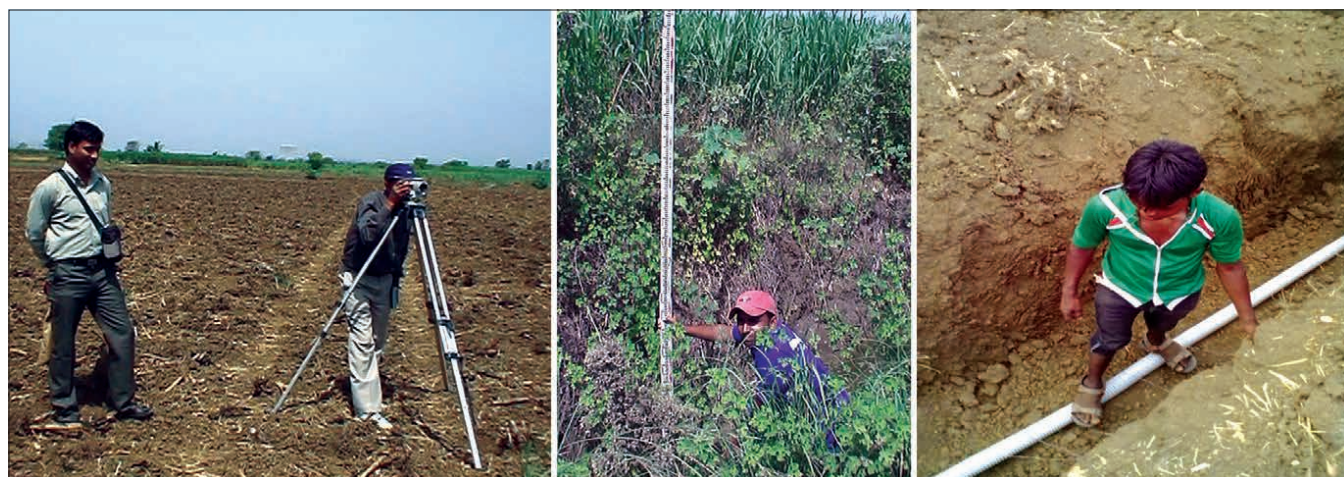
Fig. 1. Installation of sub-surface drainage
