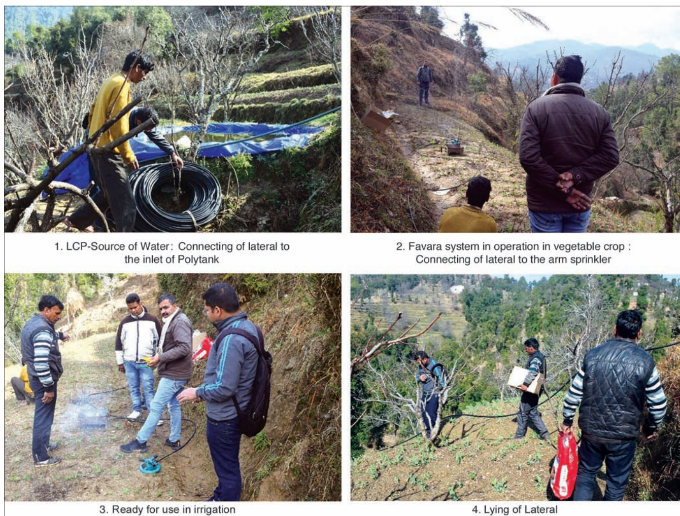
Fig. 2. Step by step (1 to 4) process for installation of GLCF
