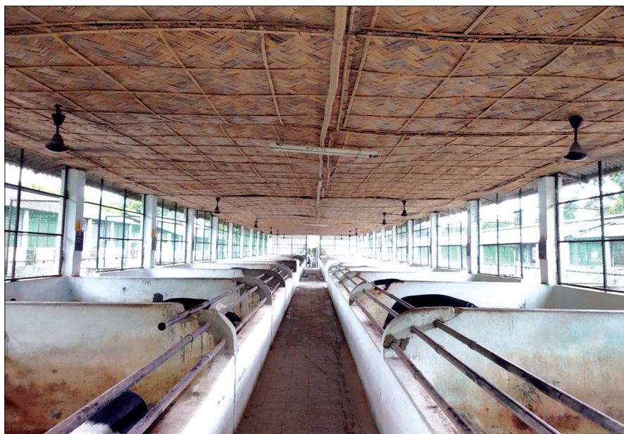
Fig. 2. Bamboo mat ceiling, fans and improved cross ventilation can reduce temperature inside pig houses
