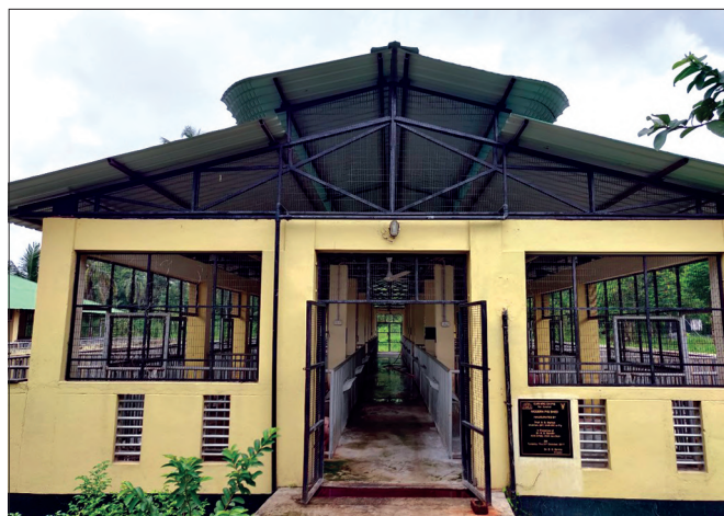
Fig. 4. Roof, wall structure and slots improve cross-ventilation inside pig houses
