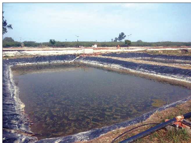
Fig. 2. Farmers found using HDPE lining in the ponds with high seepage
