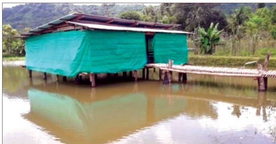
Poultry shed constructed
