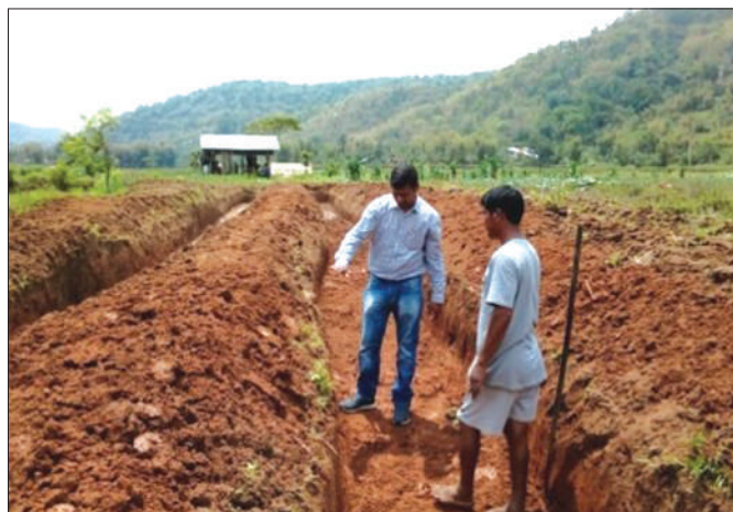
Construction of raised and sunken beds
