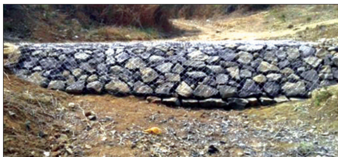
Low cost Gabion structure.
