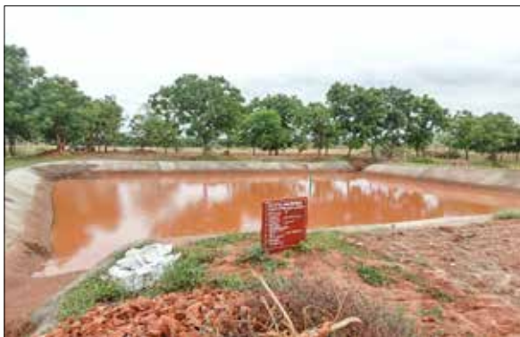
Farm pond lining with sand: cement (6:1) in scarce rainfall zone, Andhra Pradesh
