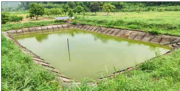
Concrete lining (5 cm thick) with bricks, Kandi region, Punjab
