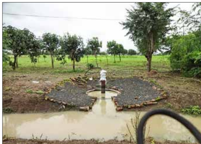
Artificial well recharging model for bore wells
