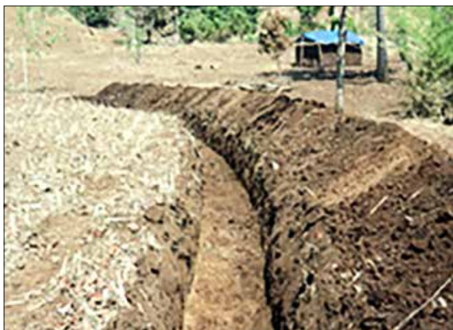
Contour trenching and bunding at Mon, Nagaland
