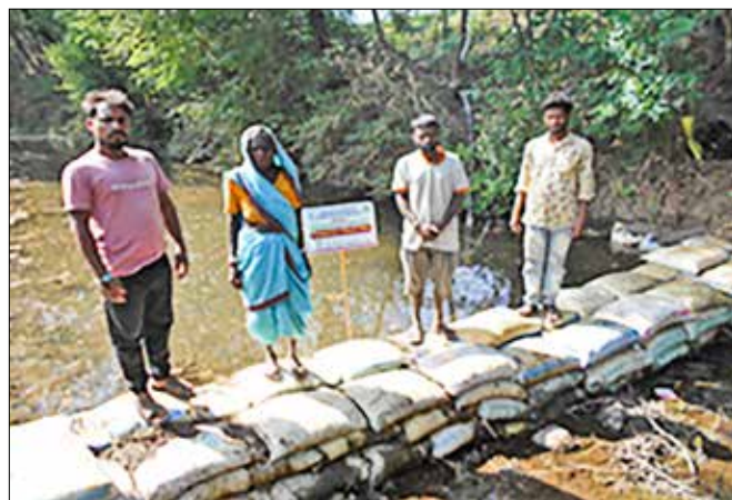
Harvested water through sand bag check dam at Nandurbar, Maharashtra
