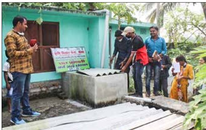
Roof top rainwater harvesting structure in Banka
