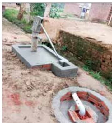
Soak pit water harvesting methods in Banka
