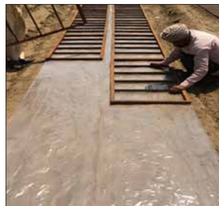
Laying of polythene sheet and iron frames
