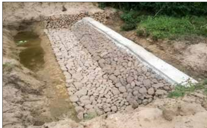
Gabions for controlling gully erosion
