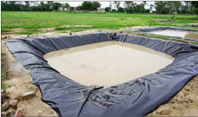
Farm ponds lined with 750 \mu polythene in Udaipur (Rajasthan)
