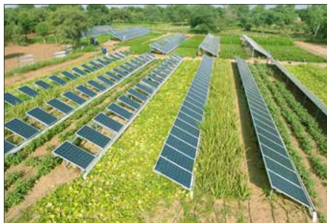
Agri-voltaic system at CAZRI, Jodhpur
