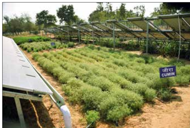
Rain-water harvesting provision on the PV panels
