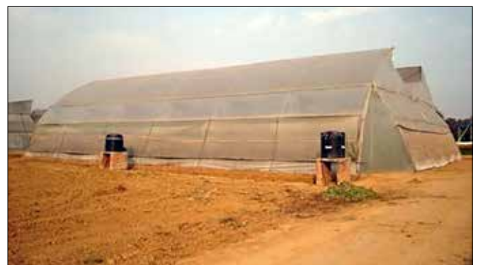
Protected structure: Naturally ventilated polyhouse
