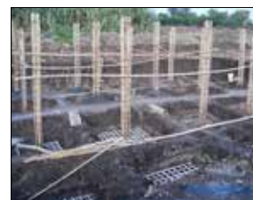
3 (Bamboo in house construction)
