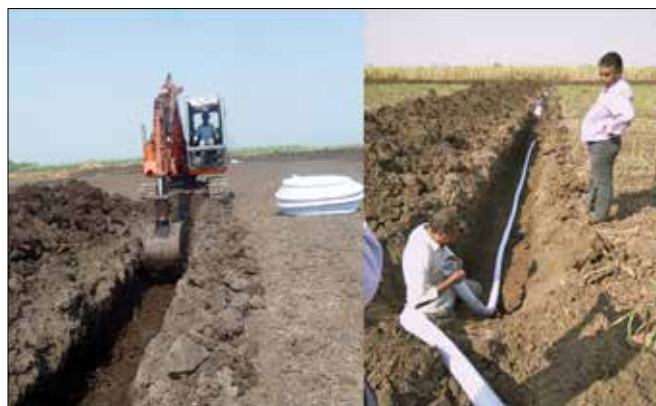
Semi-mechanized installation
