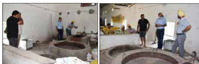
Installation of 3 pan heating system for sugarcane juice heating
