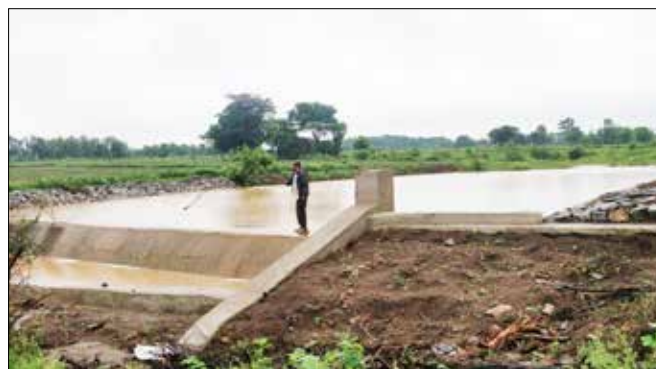
Renovated check dam in Gangupally village
