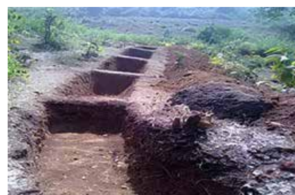
Water absorption trench
