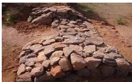
Loose boulder check dam
