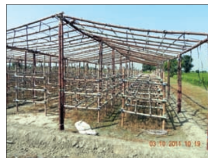
Fig. 3. Three-rack arrangement in a shed
