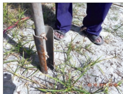
Fig. 6. Indigenous equipment to make holes in the land for shed construction
