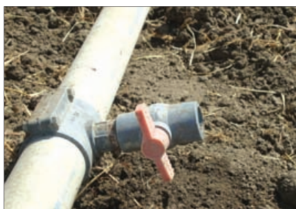
Figs. 10 and 11. Each Valve system in main pipe line to be delivered in each border - flow can be regulated using valve
