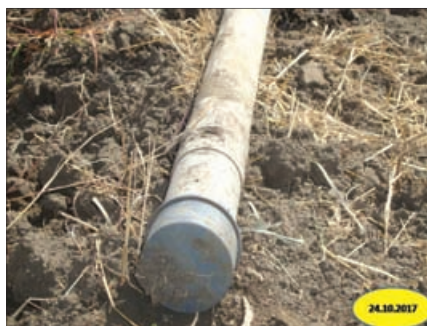
Fig. 8. End of the main pipe line tightly closed using a cap
