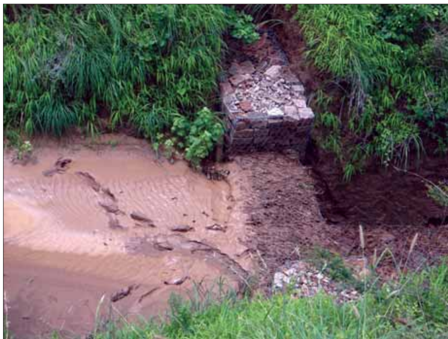
Fig. 4. Control of run-off through anicut in gully
