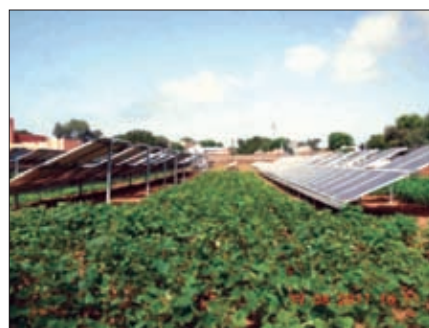
Fig. 7. Agro-voltaic system having solar panels and crops grown in inter-panel space
