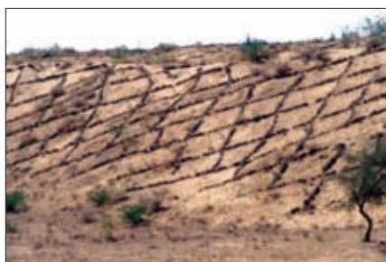
Fig. 4a. Sand dune stabilization model: Checkerboard pattern
