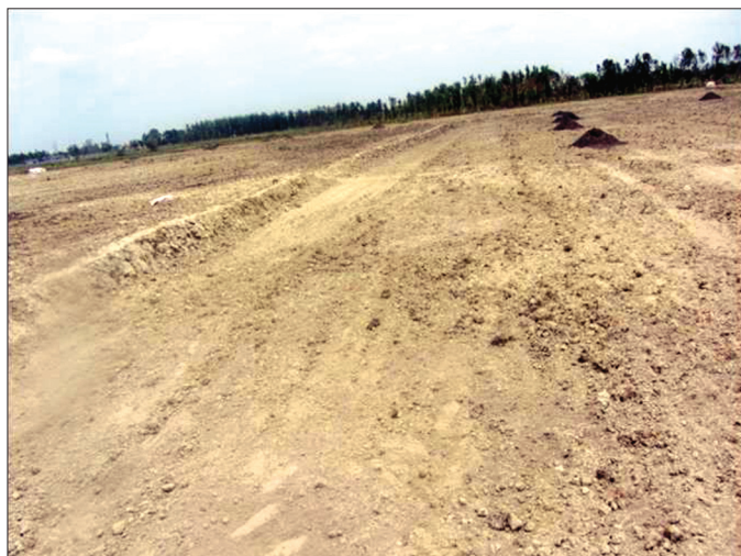
Mixing of gypsum in the surface layer
