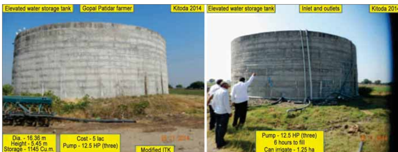
Figs. 7 and 8. Modification of traditional system of pond/talab for irrigation through gravity.
