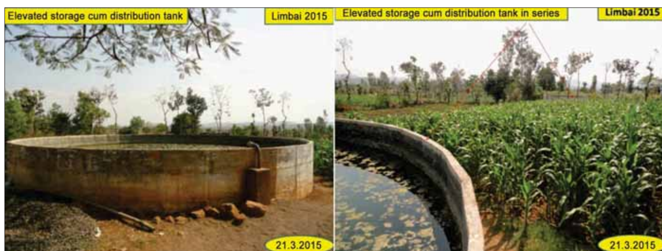
Figs 11 and 12. Elevated cement tanks in series filled with water from the gullied portion for irrigating crops in adjoining fields by gravity using micro irrigation system
