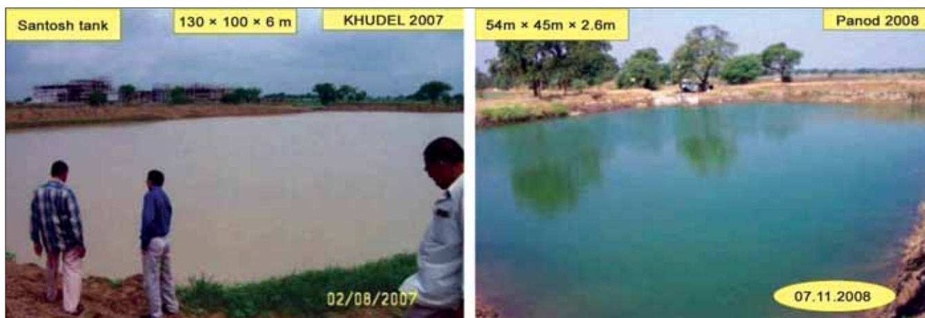
Figs 5 and 6. Construction of water-harvesting tank in the lower most portion in the cultivated field
