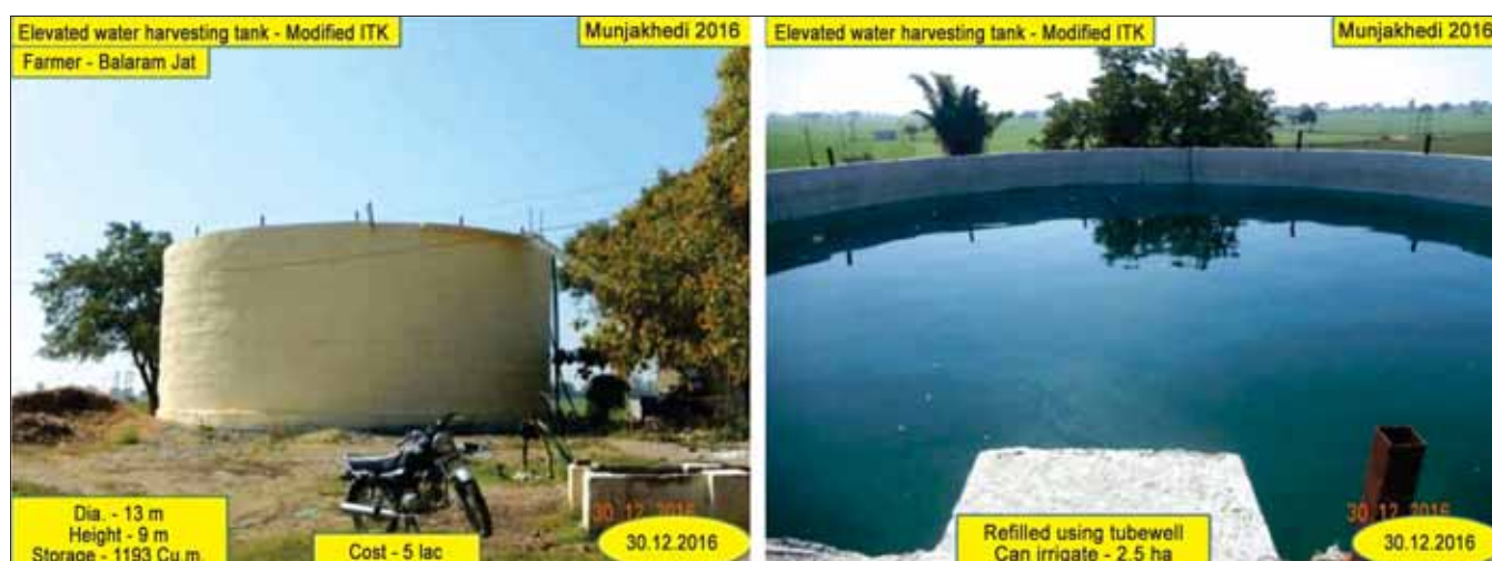
Fig. 9 and 10. Modification of traditional system filing of pond/talab with tubewell water
