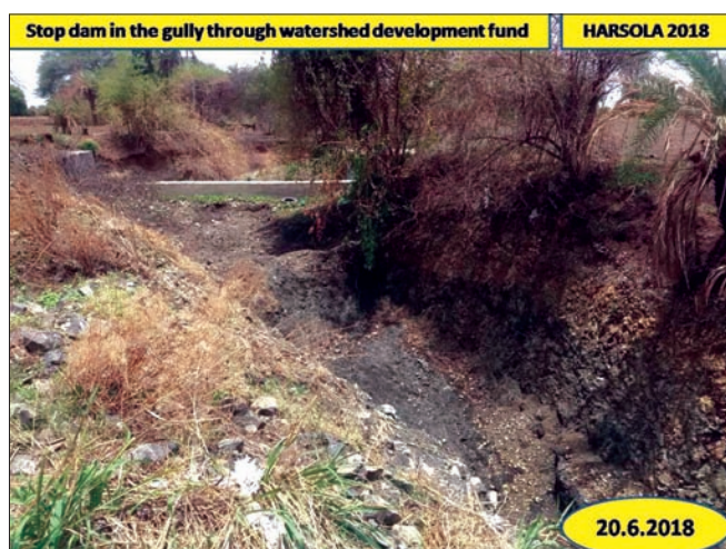
Fig. 1. Stop dam in gully where Sunken pond was created
