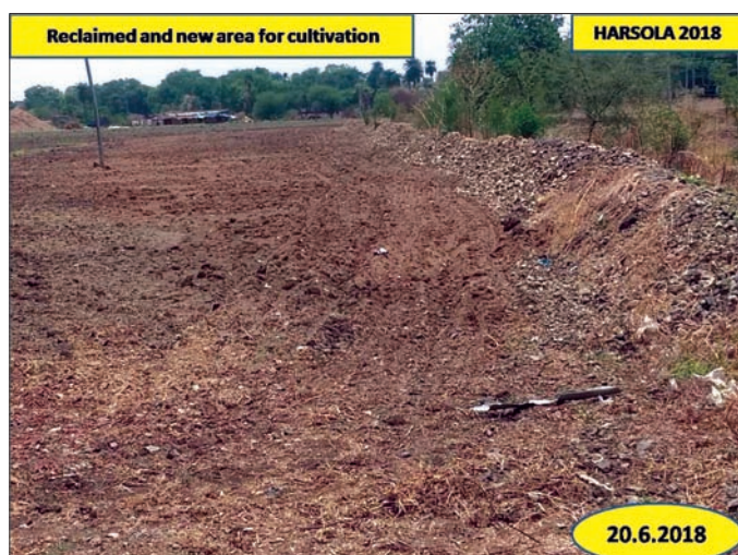
Fig. 3. Excavated soil reclaimed new era
