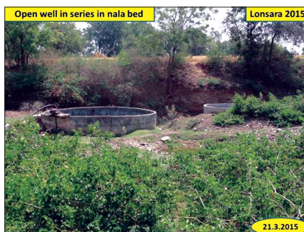
Groundwater available within 2-3 m in open well due to percolation or seepage
