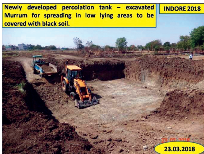
Construction of percolation tank
