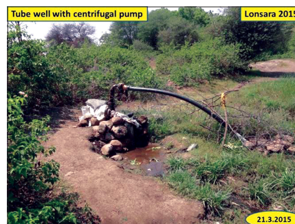
Recharged tube well use of centrifugal pump in place of submersible pump
