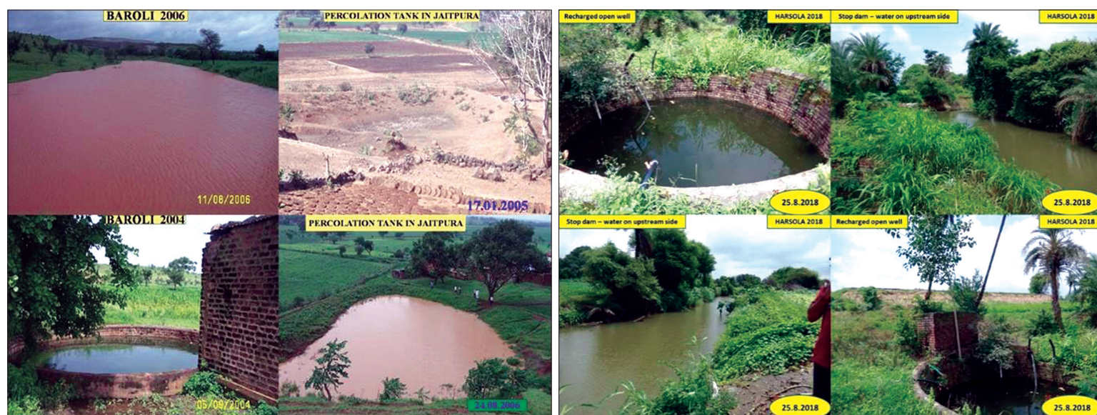
Percolation tanks adjoining to ridgeline and recharged open well
