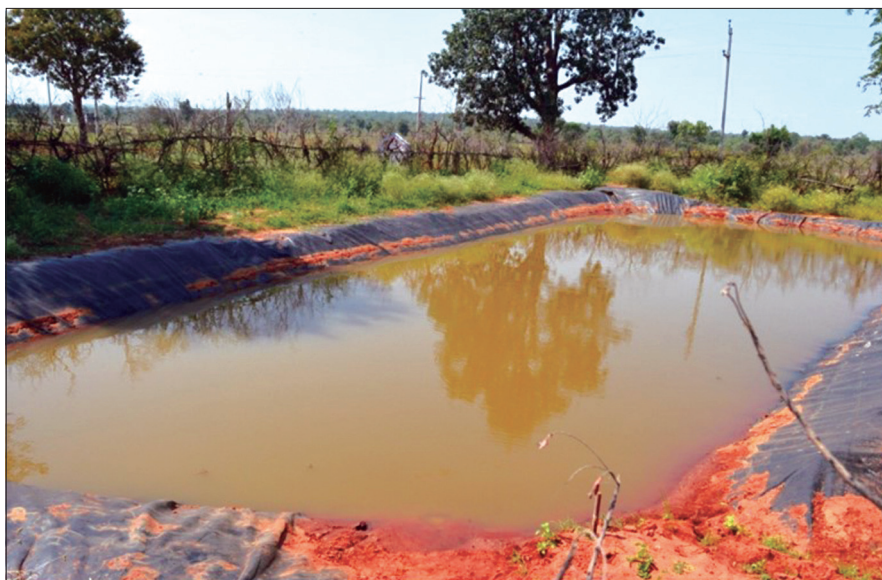
OFR with capacity of 600 m 3
