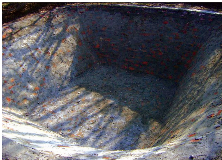
LDPE brick lining farm pond for runoff harvesting at Kulgam
