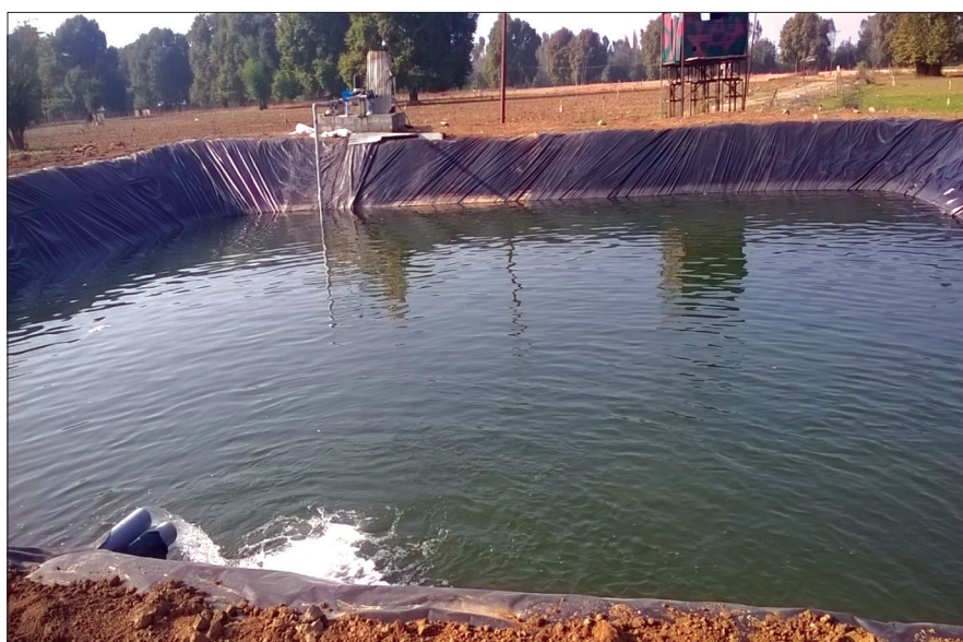
LDPE farm pond for runoff harvesting at MLRI, Mansbal, SKUAST-K
