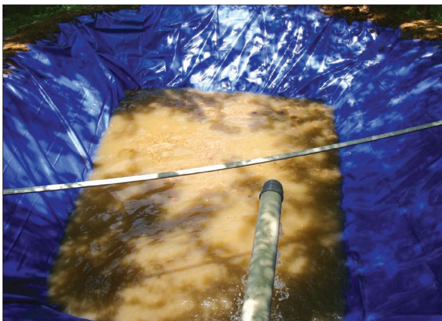
LDPE farm pond for spring harvesting at Shalimar, SKUAST-K
