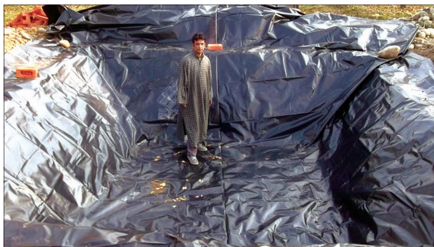
LDPE farm pond for spring water harvesting at Kulgam
