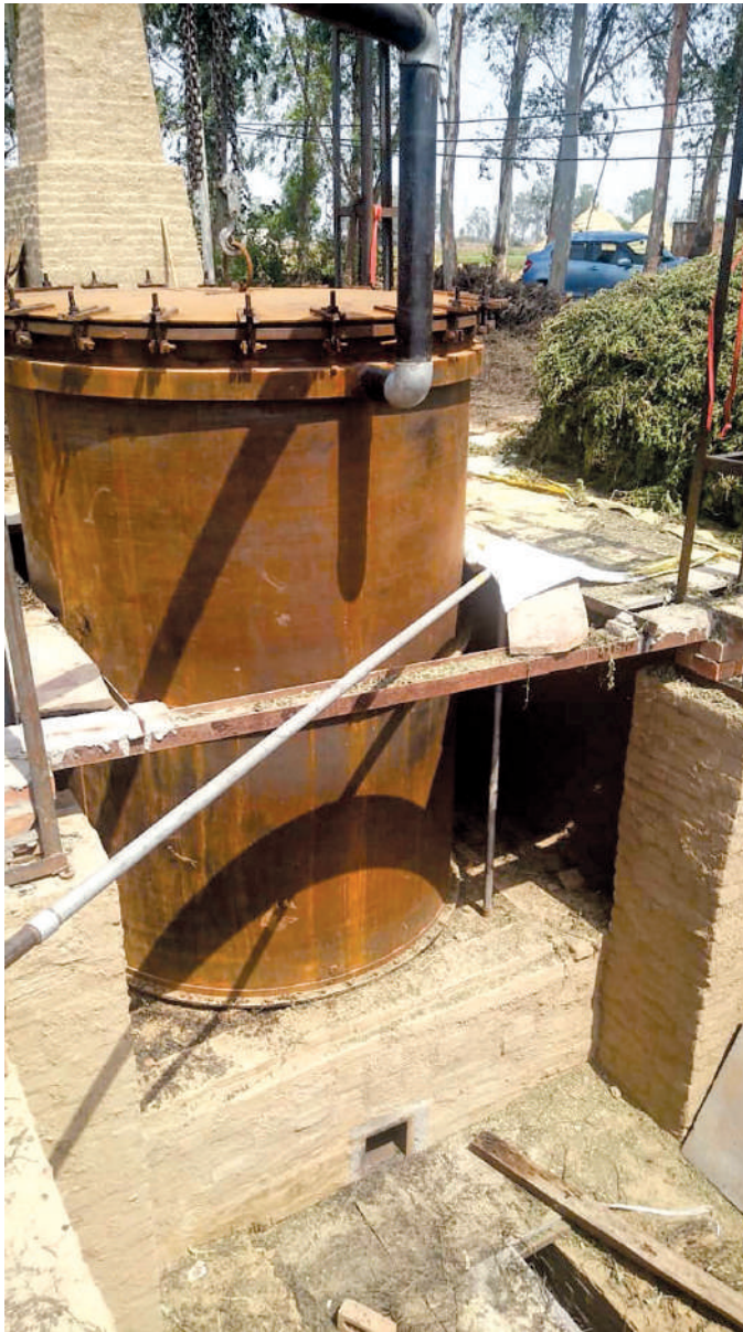
Distillation units for extracting mentha oil
