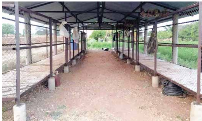
Onion storage structure
