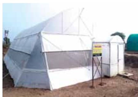
Natural ventilated polyhouse
