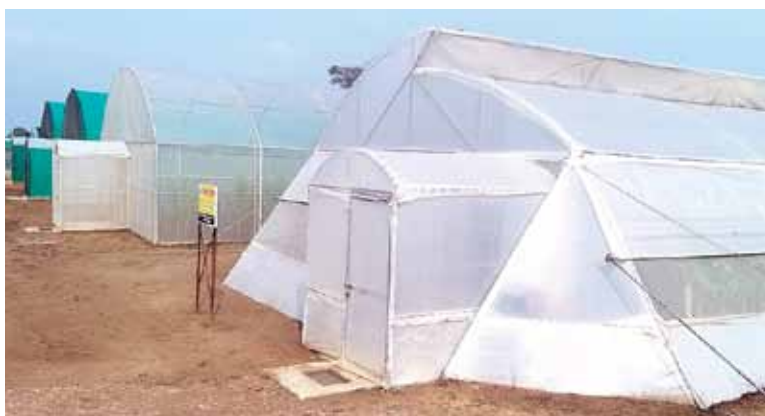
View of protected structure at BUAT, Banda
