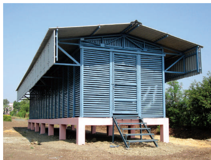
Bottom and side ventilated double row onion storage installed at ICAR-DOGR, Pune
