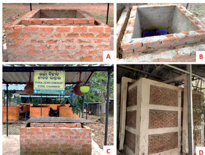
(A-C) Pusa ZECC adapted by KVK, Sundargarh-1 (Odisha); (D) Model structure of Pusa ZECC installed at ICAR-IARI, New Delhi
