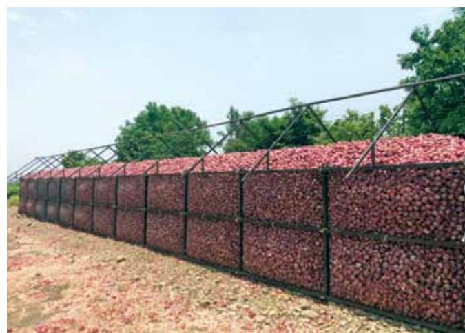
Fig. 3a. Placing of arches on the structure
