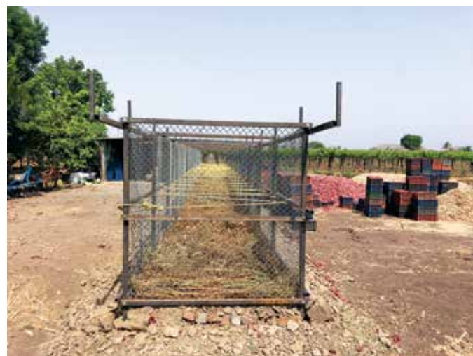
Fig. 2. Inter-connected of structure using MS pipes
