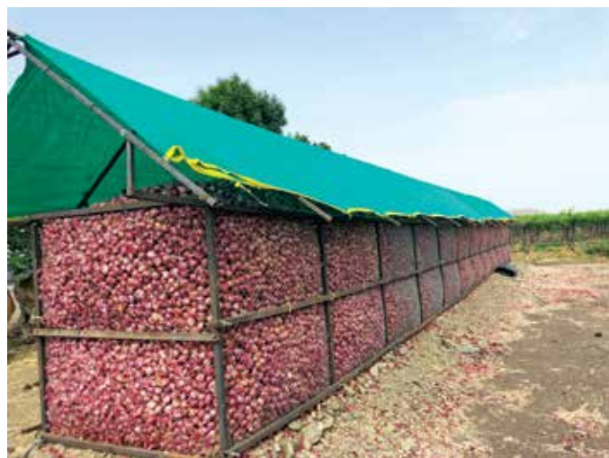
Fig. 3b. Structure is covered with shade net
