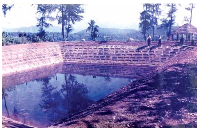
Water storage tank
