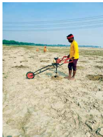
Pit preparation by Trolley Earth Auger
